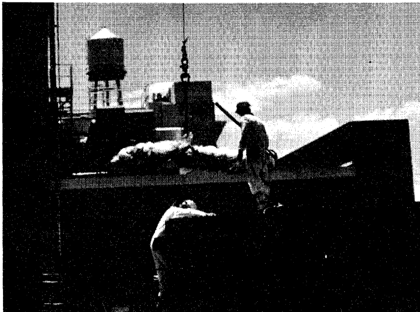
The entire recirculation piping system from the Monticello nuclear power plant (Minn.) is shown as a 12-inch riser is being unloaded to undergo both non-destructive and destructive testing at the Pacific Northwest Laboratory.
